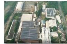
Solar Plant 1.3 MWp at M/s Timken
