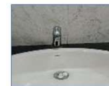
Sensor-based taps at M/s FFPL
