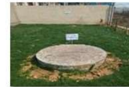
Rain Water Harvesting at M/s FFPL
